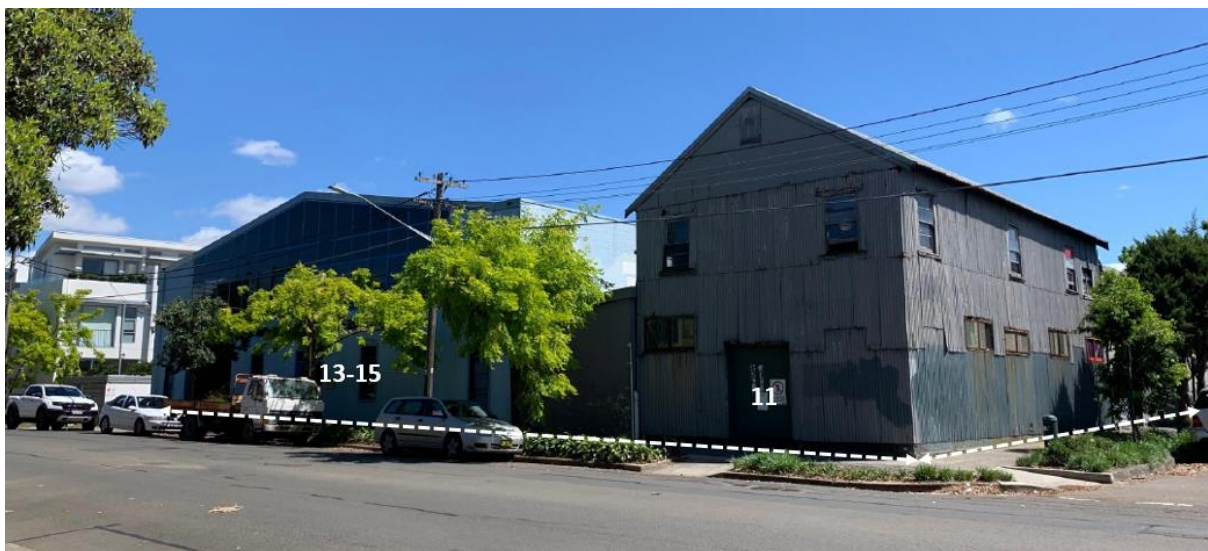
Figure 2: Site viewed from Collins Street, generally looking north-west.
