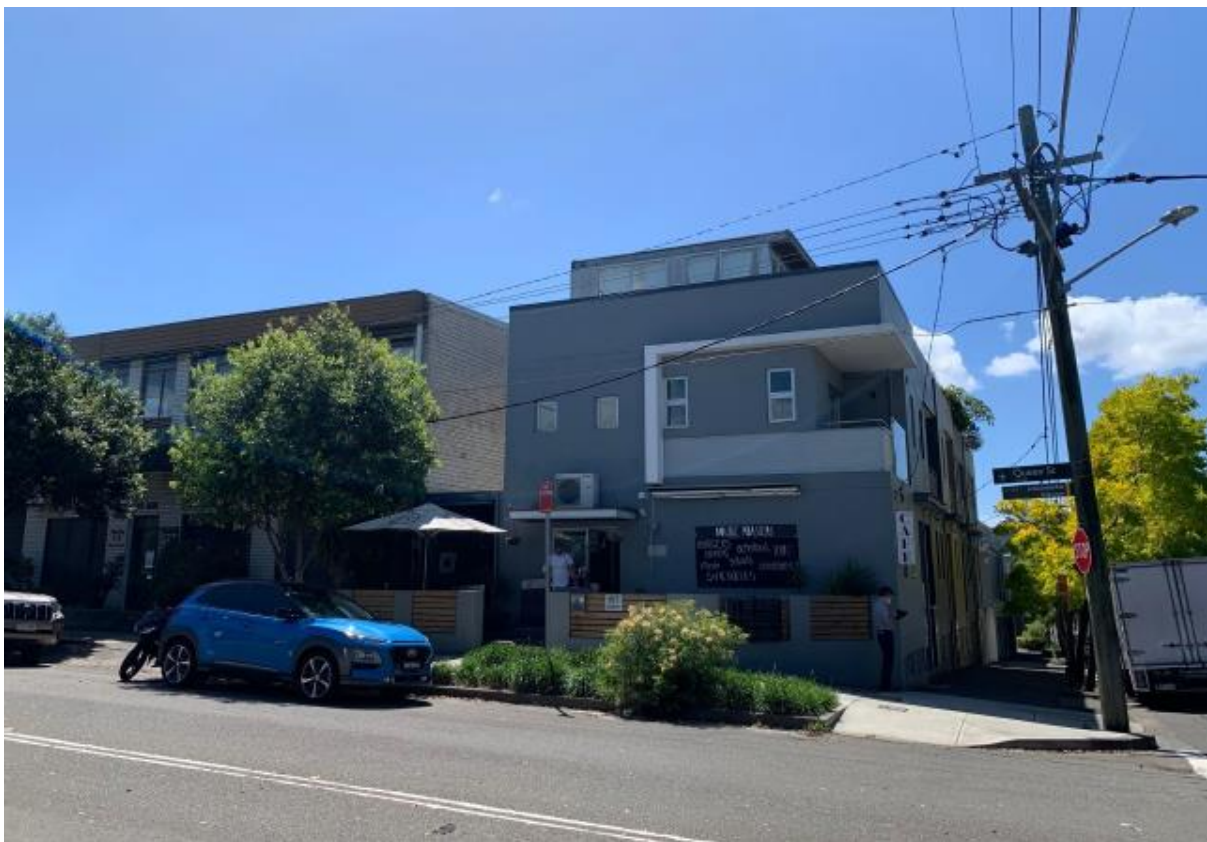
Figure 12: Mixed use development located east of the site (157 Queen Street and 9A-9D Collins Street), looking east.
