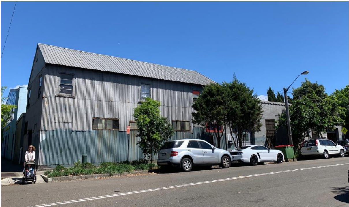
Figure 4: No. 11 Collins Street (southern end), looking west from Queen Street.
